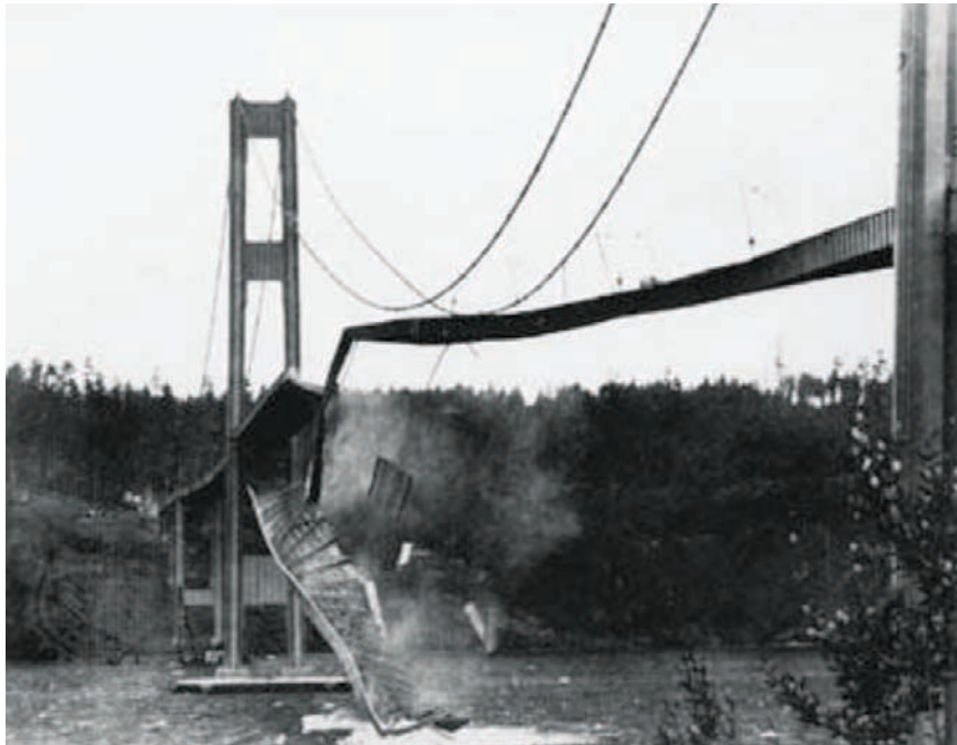
https://en.wikipedia.org/wiki/Tacoma_Narrows_Bridge_(1940) Collapse of Tacoma Narrows Bridge due to bad engineering design and poor engineering skills in order to provide the reliable design.
